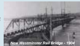
New Westminster Rail Bridge - 1904
